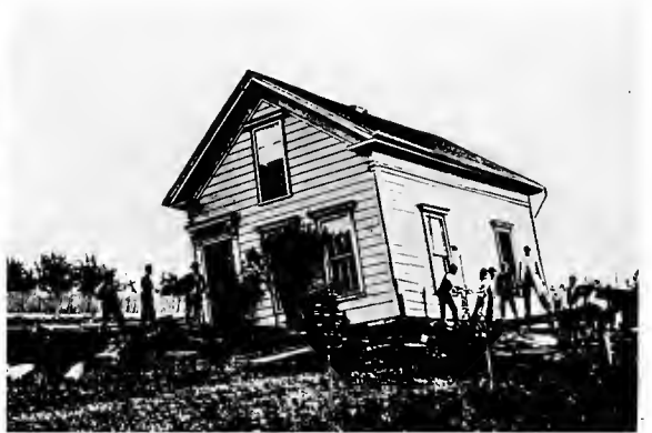
D. Pierce's house, Haywards. Earthquake of 1868.
